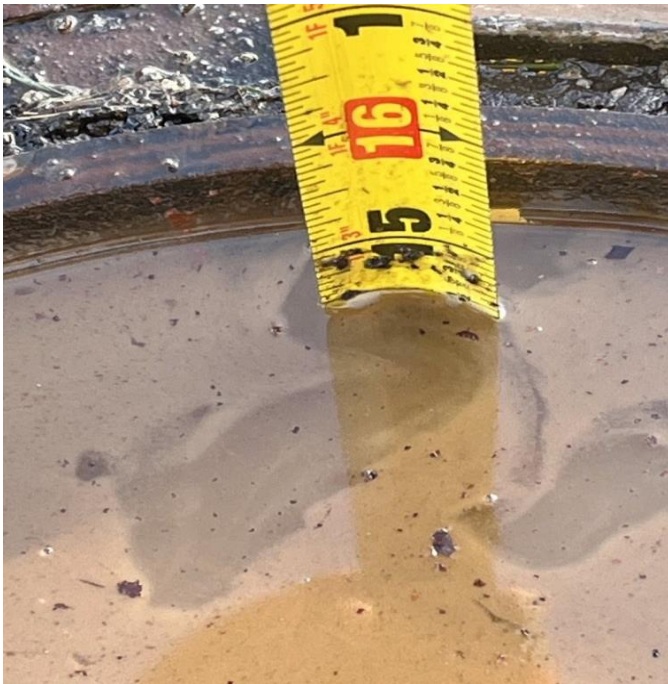
KER SPILL BUCKET TEST START 14.5"
