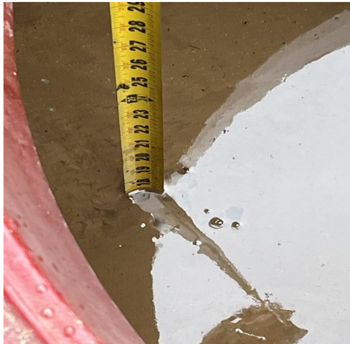
DSL STP SUMP TEST END 17.75"
