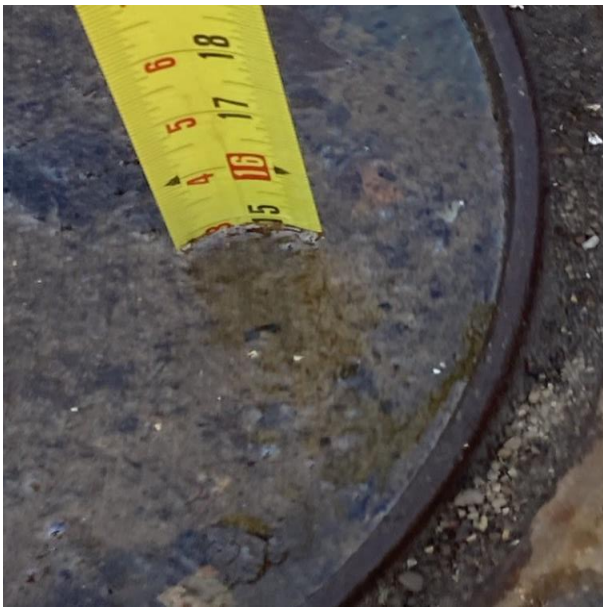
PUL SPILL BUCKET TEST START 7.5"
