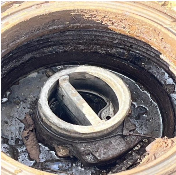
RUL2 - UNABLE TO REMOVE DROPTUBE
