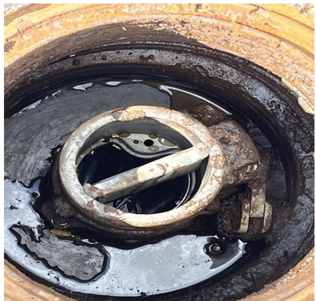
RUL1 - UNABLE TO REMOVE DROPTUBE
